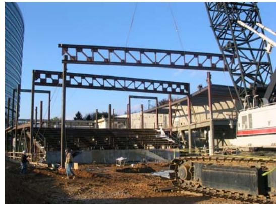
Figure 10. Placement of Steel Trusses
