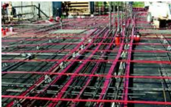
Figure 6: Typical tendon layout. Taken from www.concreteconstruction.net
