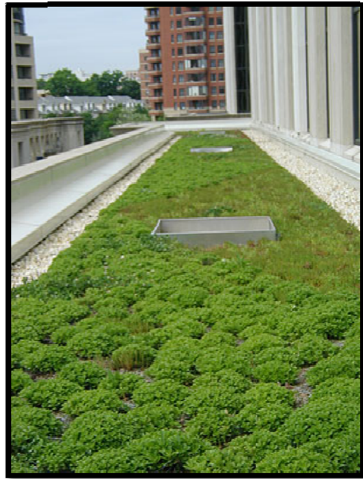
Figure 4 Typical Green Roof System
