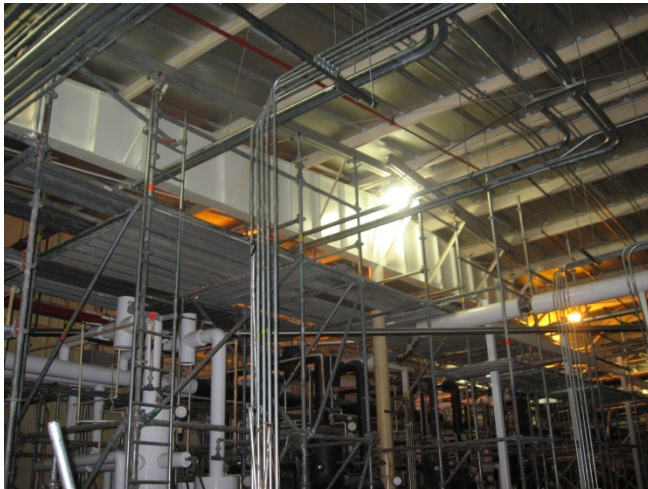
Figure 1, shows the repairs made to structural frames.
