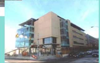
11/28/07 – Precast finished at southwest corner
