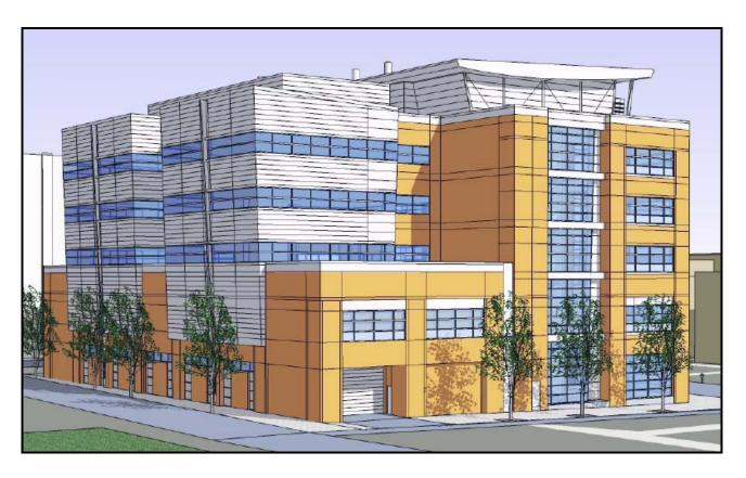
The Forensic Medical Center is a five-story, 105-foot tall building, with 121,000 square feet of office, classroom, and laboratory space. The structural system as designed is an 11"-thick two-way flat-plate concrete slab, with 24"x24" concrete columns, and a dual lateral system consisting of concrete moment frames and 12"-thick concrete shearwalls.
