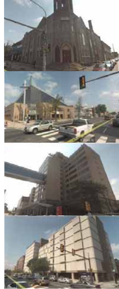
Residential buildings, above – Campus buildings below.
