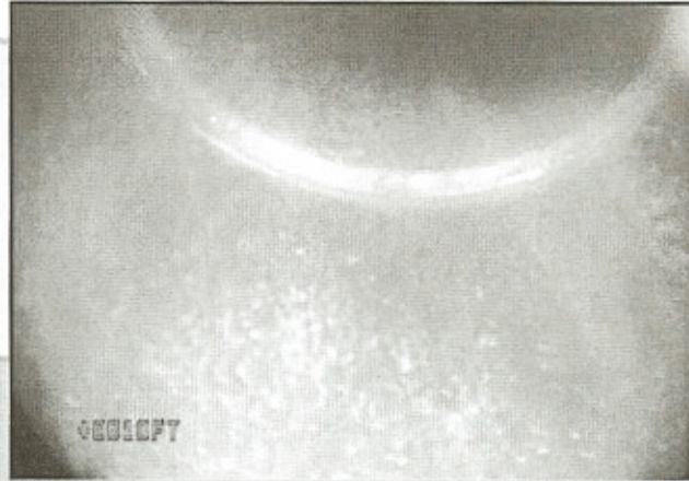
Casing joint not completely shouldered
