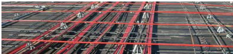
Figure 9: Vertical Tendon Layout
