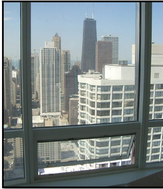
Figure 4: Open Operable Window Facing Down at Floor Level in Trump Tower
