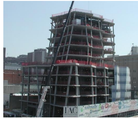
Figure 7: Flat plate system during construction of the IAC Headquarters
