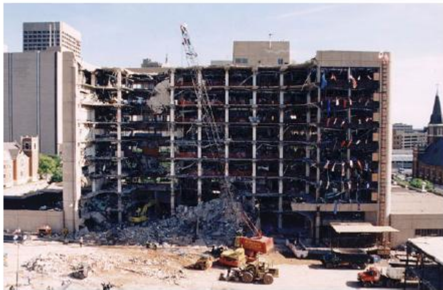
FIGURE 9 – Murrah Federal Building after bombing (FEMA Primer 2003)
