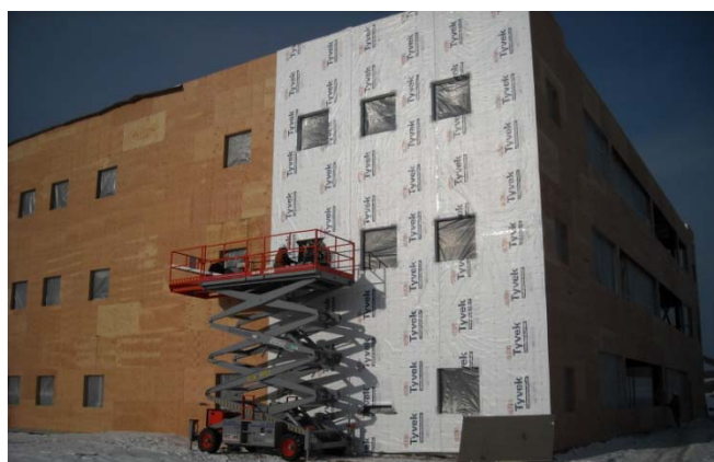
Figure 5: Installation of the Tyvek wrap
