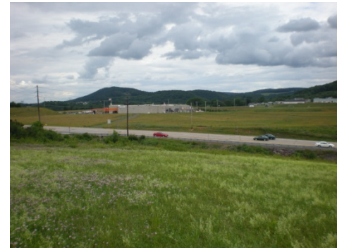
Figure 1: The existing site before excavation
