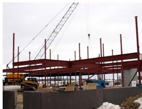
Figure 3: Steel erection during winter months
