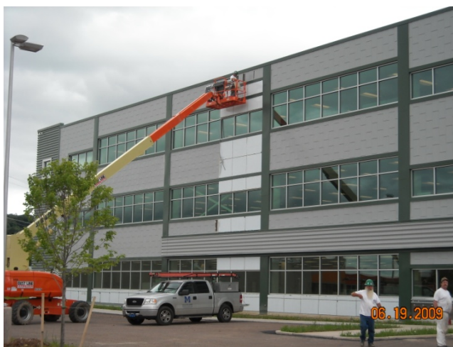
Figure 10: Installation of the aluminum panel system
