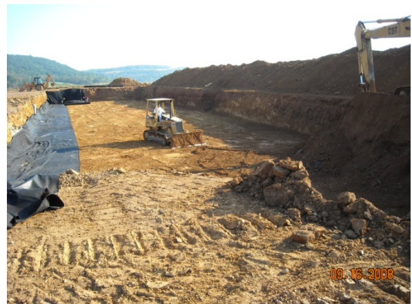
Figure 2: Excavation for the foundation of the building
