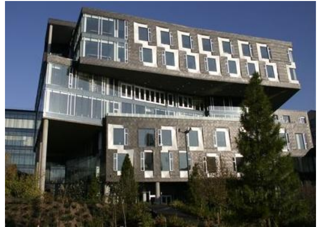
Figure 41- West elevation showing the use of windows
