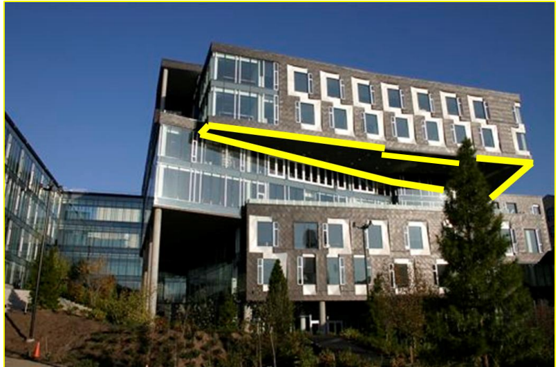
Image 23: Image of west façade with highlighted cantilever
