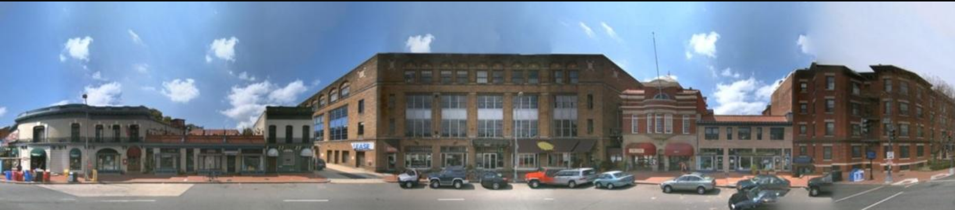
Located on the U Street Corridor: D.C. Historic District
