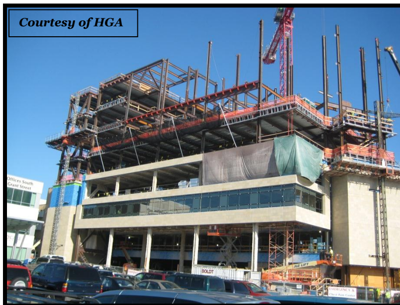
Picture 4: Construction of the addition
