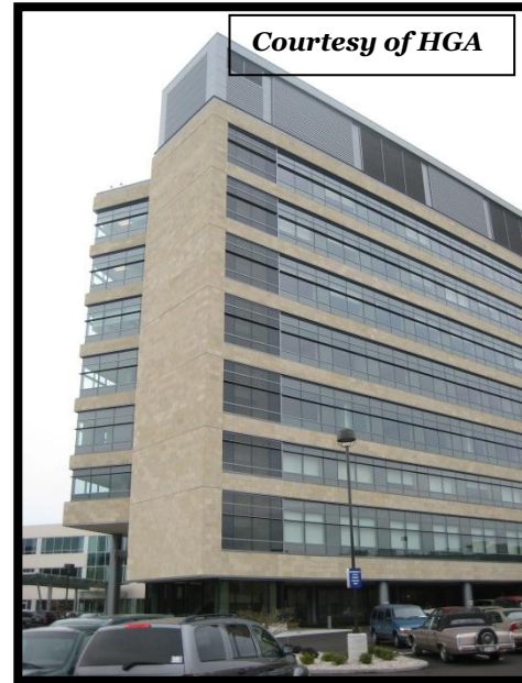
Picture 3: Bed Tower Addition
