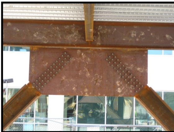
Figure 3: Close-up of gusset plate construction for the braced frame
