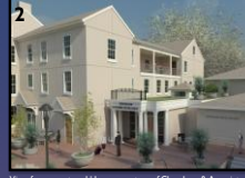
View from courtyard | Image courtesy of Chambers & Associates
