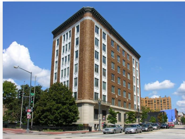
Figure 3-1: Image of Existing Building
