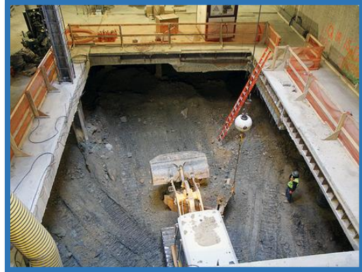
Figure 7: Top-Down Excavation
