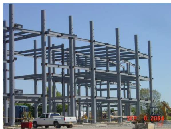
Figure 6 | Photograph during erection of HSS framing
