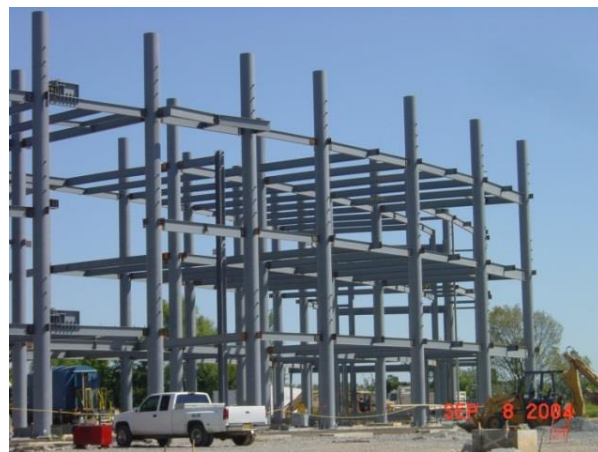
Figure 6 | Photograph during erection of HSS framing
