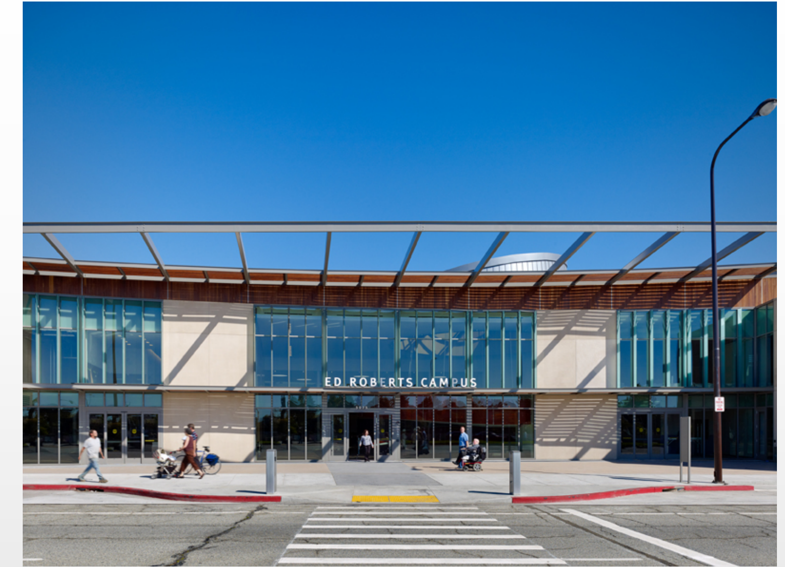
Leddy Maytum Stacy Architects, Photo by Tim Griffith
