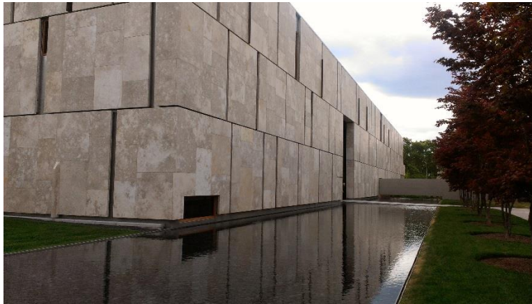
Figure 1 | Exterior Walkway | Courtesy of FMS
