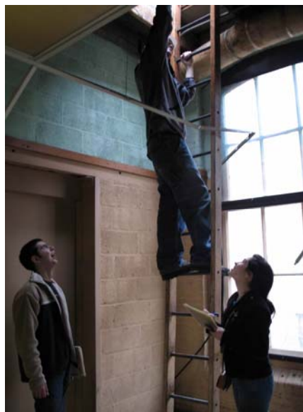
FIGURE 4 STUDENTS EXAMINING THE CMAA BUILDING
