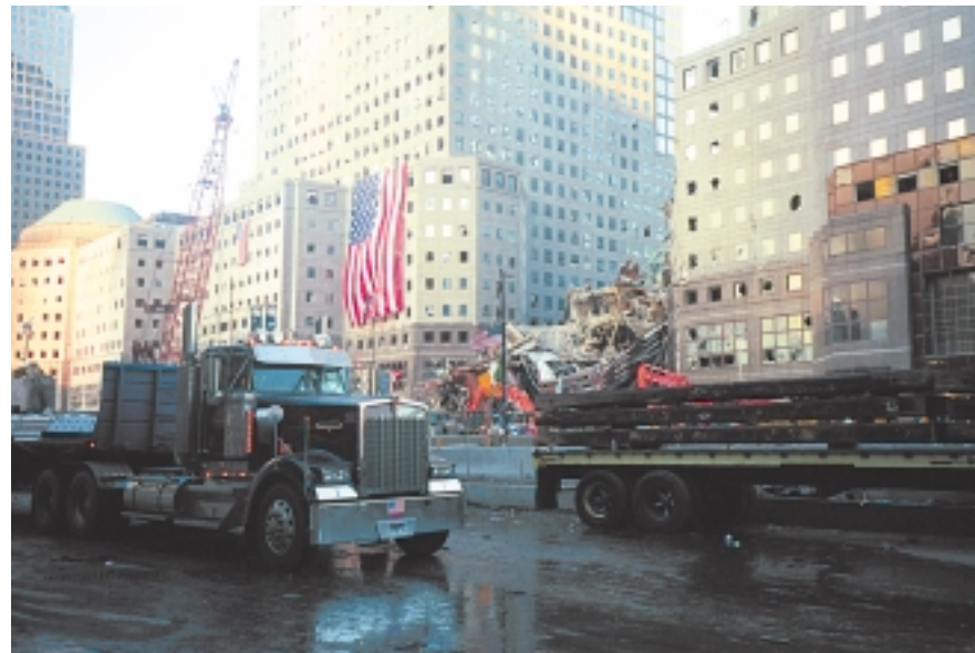
Top: Towers 1 and 2, looking south. Bottom: The World Financial Center's Winter Garden, collapsed at center.
