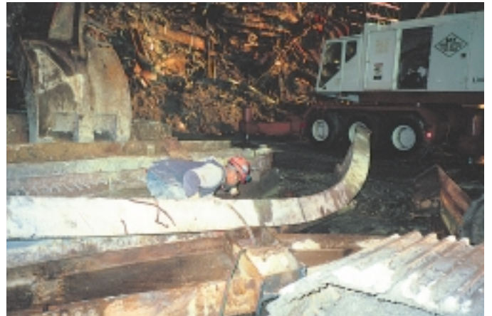
A bent W27 steel beam in the wreckage.
