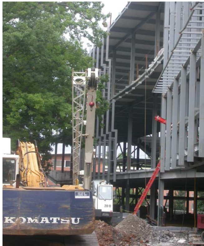
Figure 6.5: Steel trade installing tube steel due to the congested site
