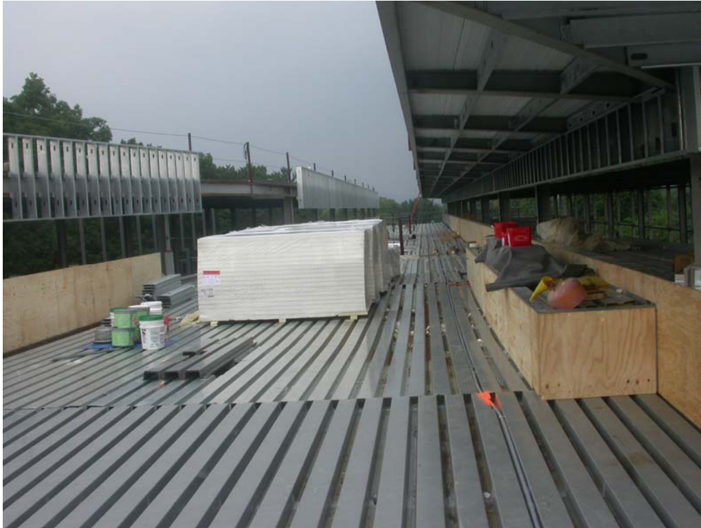
Figure 6.3: Site space condition: Material storage on the roof
