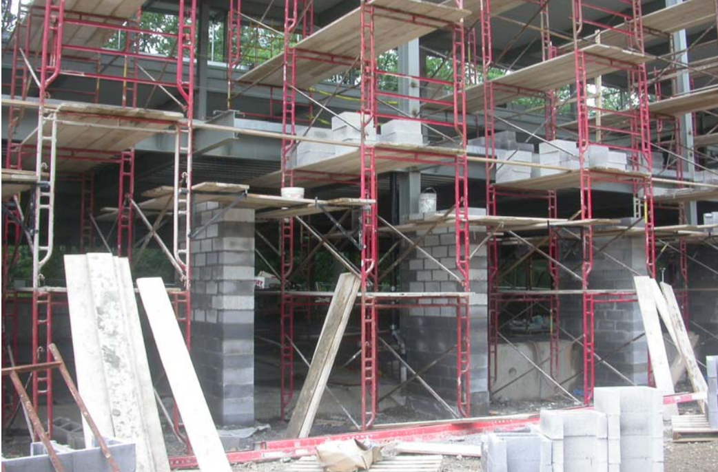
Figure 6.6: Masonry trade scaffolding for brick piers along B Line
