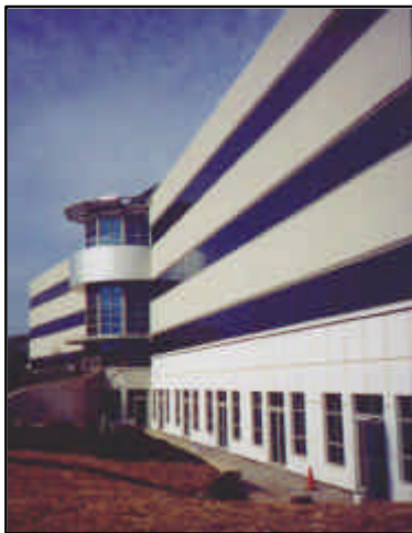
Figure 1.1 The building façade alternates EIFS panels with 4 ft. seamless mullion ribbon windows.
