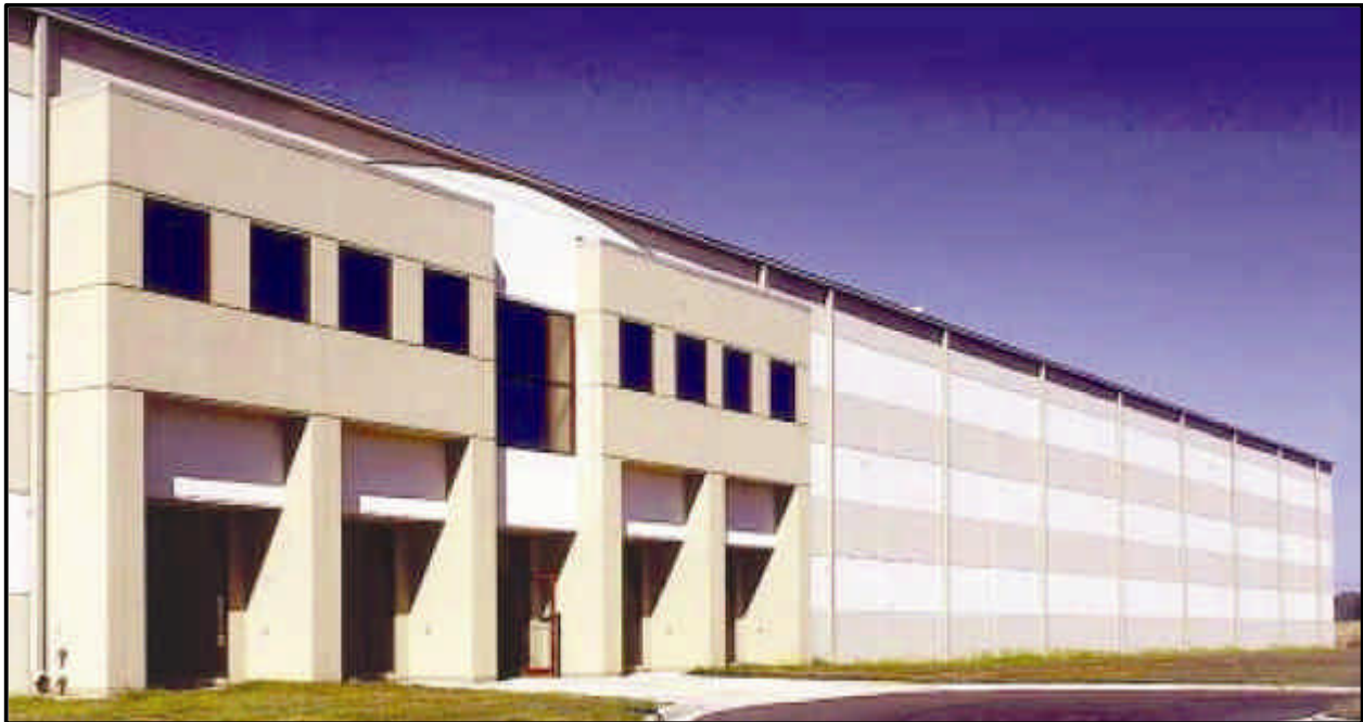
Figure 2.1 Precast concrete panel finish appearance. (Houston Co. Spec., Perry, GA – Tindall Corporation)
