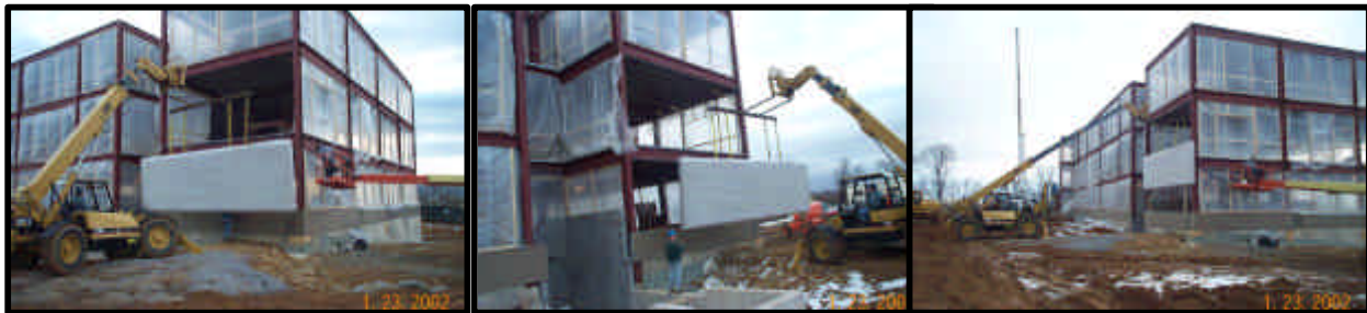
Figure Prefabricated EIFS panels were hoisted into place with a special rigging attached to a fork lift. An average of 1 panel per day was raised by this method.
