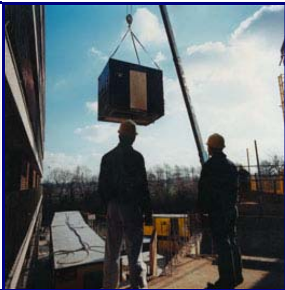
Unit Lifted into Place - http://www.modularuk.com
