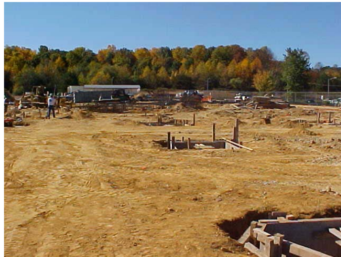
Site View prior to pouring pile caps
