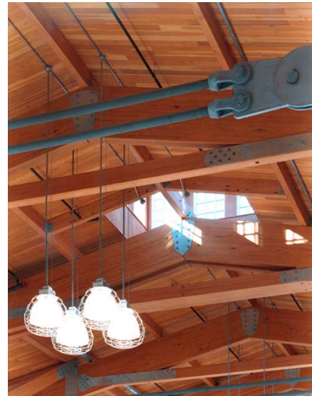
Figure 11. Truss bottom chords. Photo credit: www.som.com.
