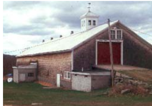
Figure 4. Cow Barn at Alfred Shaker village, includes cupola. Credit: National Park Service.
