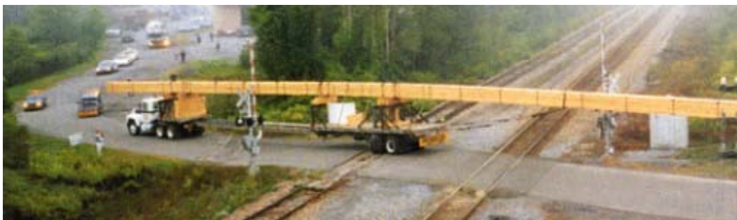
Figure 13. Unadilla Laminated Products delivering one of their beams to a site.
