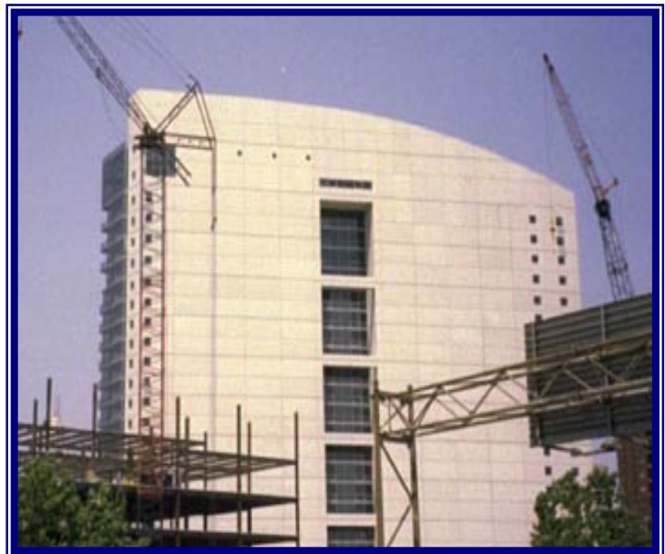
Figure 2: South Side of Building
