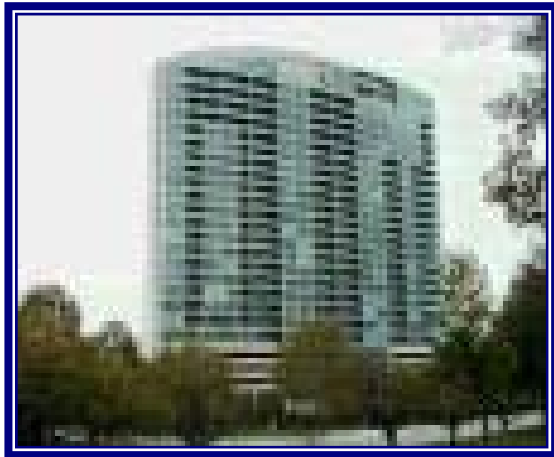
Figure 1: North Face of Building
