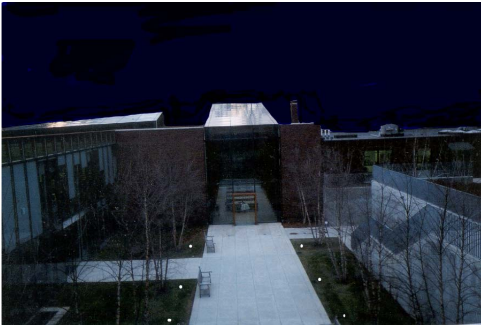
This view shows the location of the recessed uplight. The lighting levels will reflect the luminance shown here. Even lighting across most of the pavement, and high contrast points of interest in the grassy areas.
