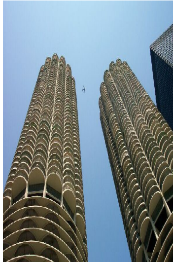
Marina City in Chicago, IL is an Architectural Concrete Structure Made Using Fly Ash
