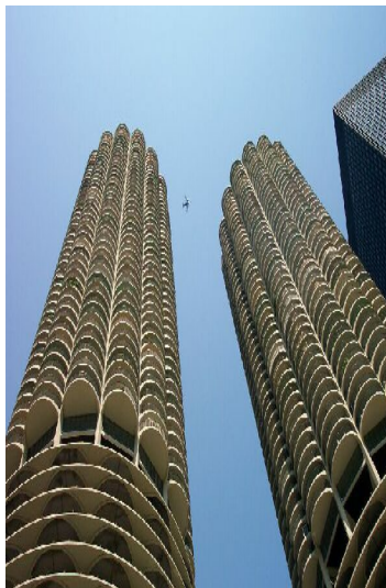
Marina City in Chicago, IL is an Architectural Concrete Structure Made Using Fly Ash
