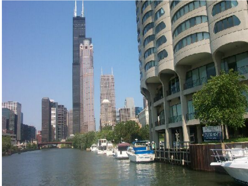
The Sears Tower and River City are Buildings Constructed with Fly Ash
