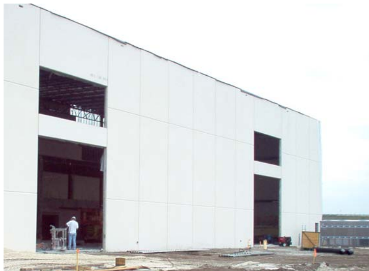
Figure 6: Concrete Tilt-Up Panels – Simulator Bay
