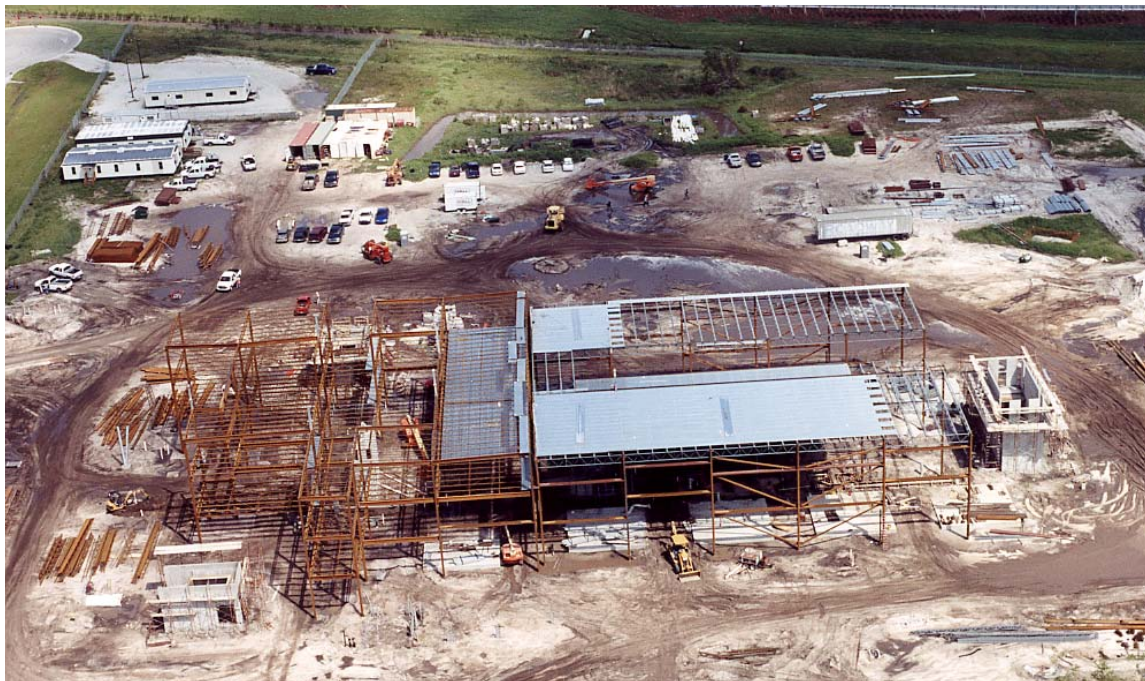
Figure 7: Structural Steel Erection
