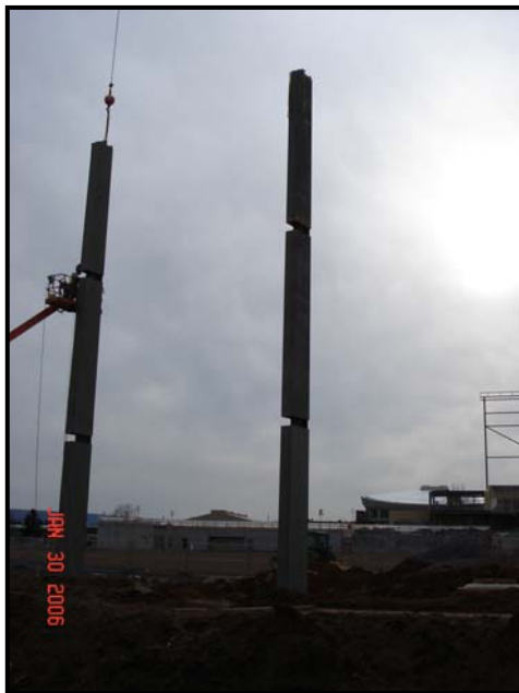
Erection of Lighting Structure Columns
