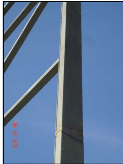
Grinded Splice Plate Connection
