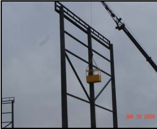
Detailing/Welding Splice Plate Connections
