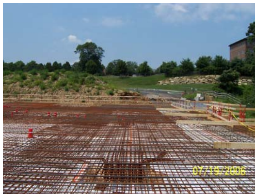
Picture 3: Foundation Columns and Footings installed prior to slab on grade
