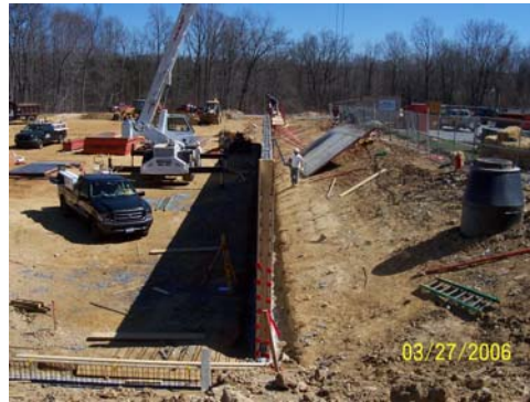
Picture 1: Column Footings being erected
