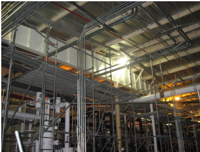
Figure 1, shows the repairs made to structural frames.
