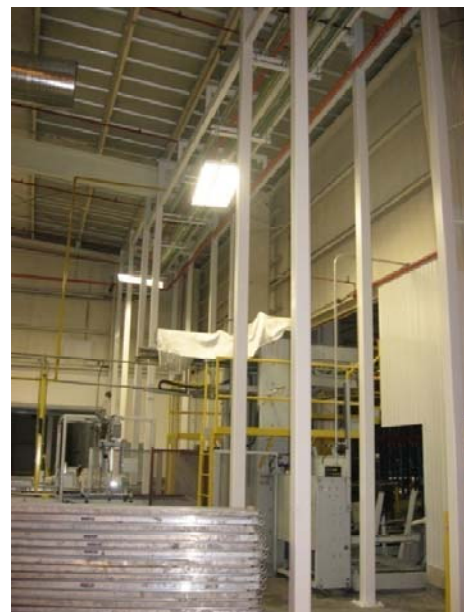
Figure 2, shows the braces that were added to remove load from the structural frames.
