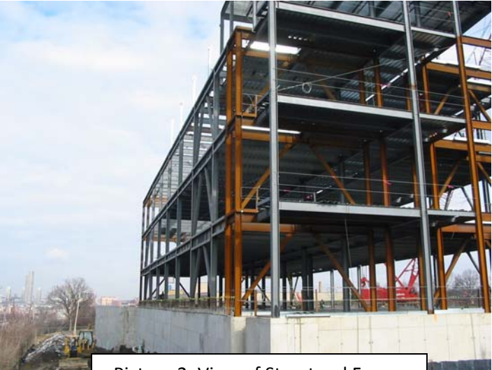
Picture 2: View of Structural Frame
