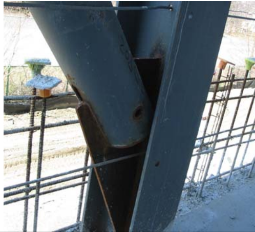
Picture 4: Typical Lateral Brace Connection
