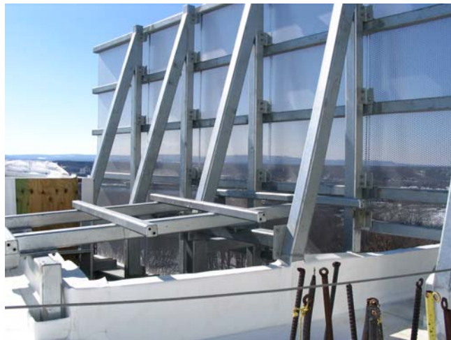
Picture 6: Penthouse Mechanical Screen
