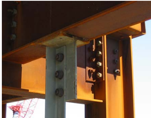
Picture 5: Typical Column-Girder Connection
