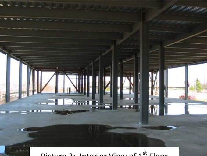
Picture 3: Interior View of 1 st Floor
