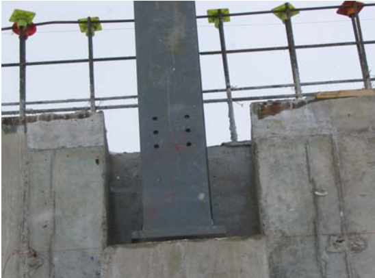
Picture 1: Typical Structural Column on Pier
