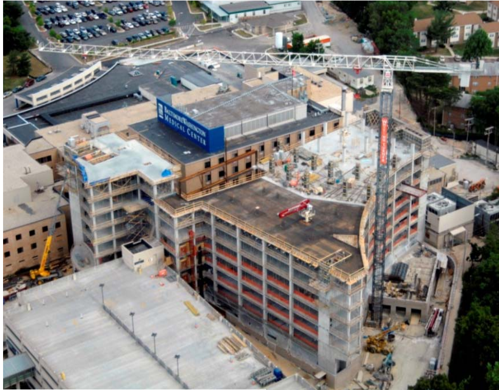
Figure 9: Construction of Patient Tower
