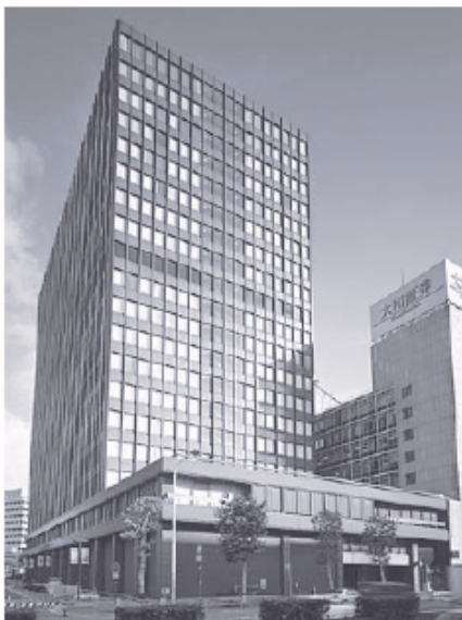
Figure 14 – Nippon Steel Building in Tokyo, Japan (courtesy of AISC)
