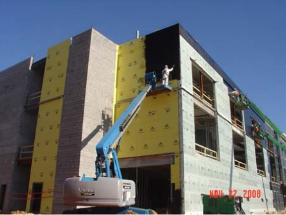
Figure 12, Vapor Barrier over Exterior Sheathing
