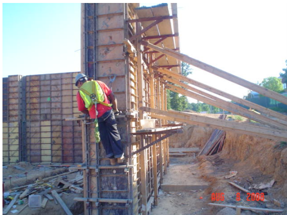
Figure 8, Support and forming of north retaining wall
