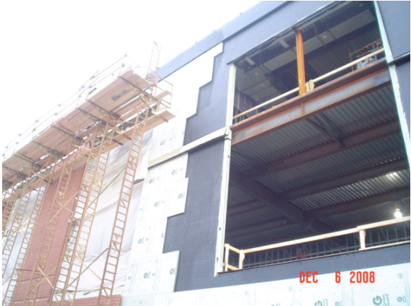
Figure 13, Brick Veneer being installed over Vapor Barrier
