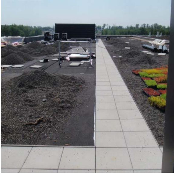
Figure 9, Green Roof Installation
