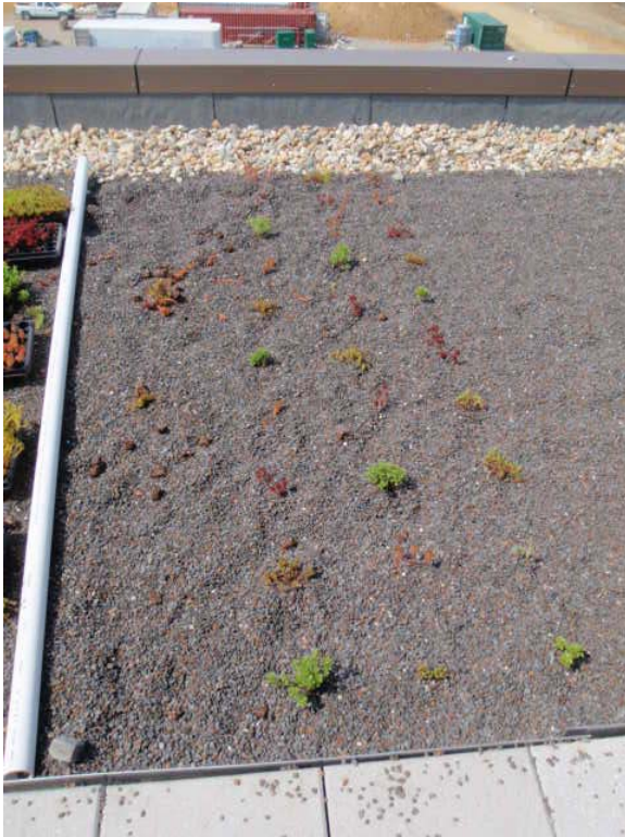
Figure 10, Green Roof Plantings
