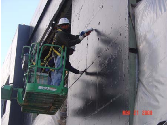
Figure 11, Installation of Vapor Barrier
