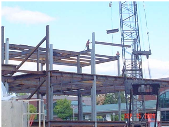
Figure 6, Steel Erection via Lattice Boom Crane
