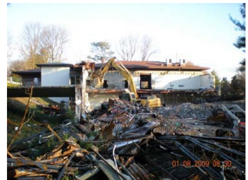
Figure 2 - Demolition of Existing Structure
