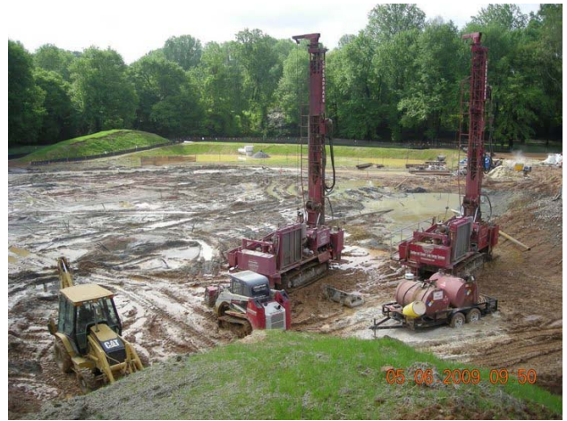
Figure 5 - Drilling Rigs in Geothermal Field
