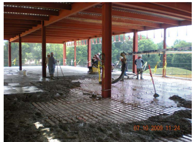
Figure 4 - Pumping Concrete to Elevated Slab
