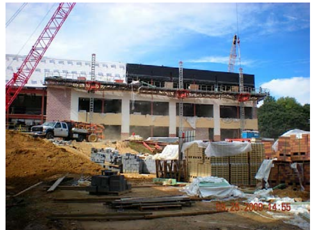
Figure 6 - Masonry Veneer and Staging Area
