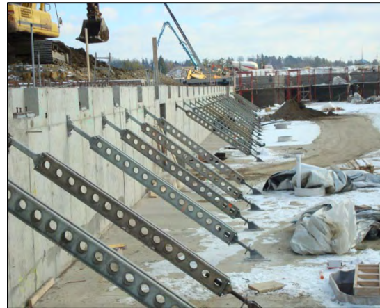
Figure 19: Recently Complete Mabey Project (Image supplied by Mabey Bridge & Shore, Inc)
