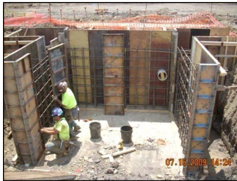
Figure 6: Mod-U-Form installation
