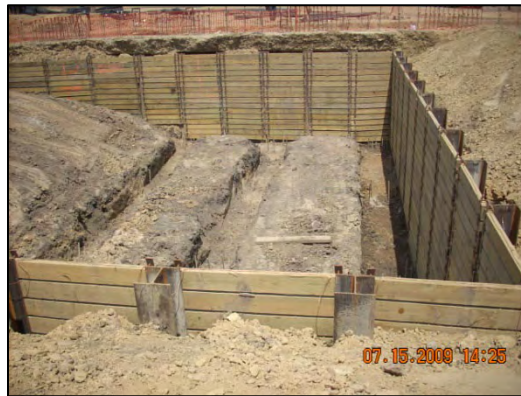
Figure 8: Supported Excavation Surrounding Pool
