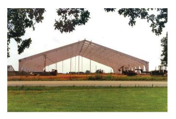
**Figure 9-1.1 - Glulam Arches** (Courtesy of Structural Mag)
