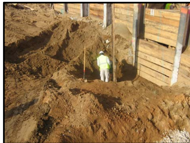
Figure 6: Support of Excavation
