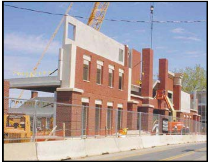
Figure 63: Brick masonry panels (The Shockey Precast Group, 2008/2009)
