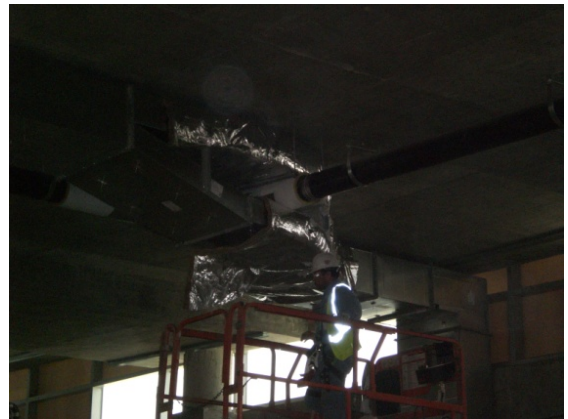
Figure 1 – 2 nd floor ductwork and plumbing clashes
