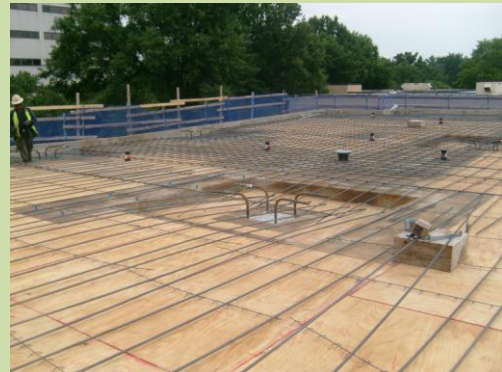
Low-roof reinforcement before slab is poured
