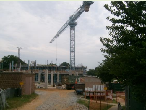
Crane Used on site
