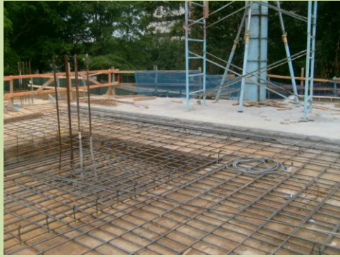
Central Park location w/ post tension Reinforcement
