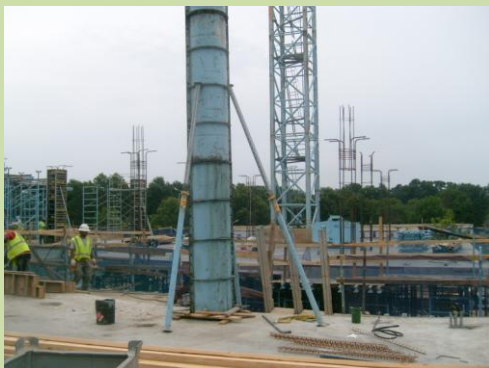
Column Formwork
