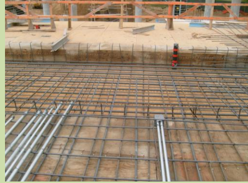
Post tensioning reinforced slab
