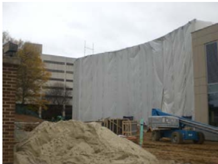
Figure 2-Temporary Building Enclosure
