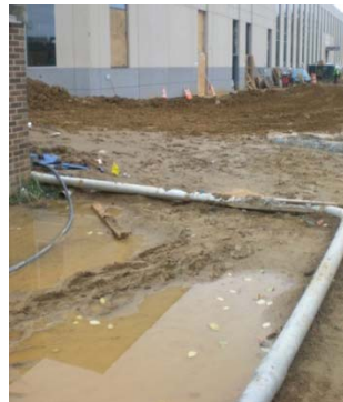
Figure 4 – Replacement of Site Utilities
