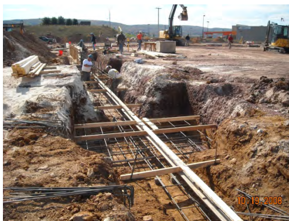
Figure 1: Foundations being place along the south wall
